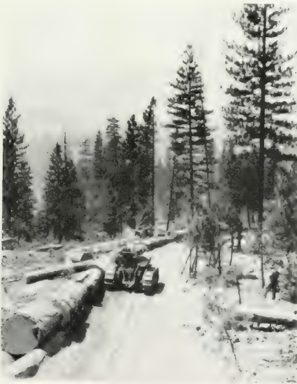
FIG. 138. CATERPILLAR HAULING TURN OF LOGS ON POLE ROAD, U.S.A.
